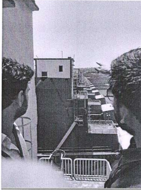
Side View of spillway
